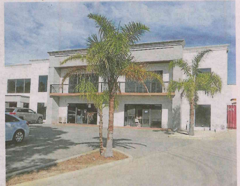
The three industrial properties are in Wangara, north of Perth.
